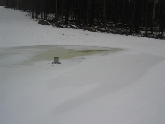
Photograph of wet pond - Town of Hague subdivision taken on January 30, 2008. Note the freeboard height of the standpipe above the ice elevation.
