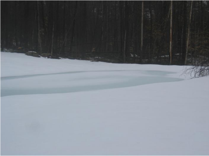
Photograph of same wet pond – Town of Hague subdivision taken on March 20, 2008. Note that there is no freeboard on the standpipe above the ice resulting in direct discharge of runoff without management or treatment.
